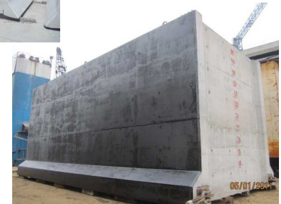
Pre-casting of Concrete u-channel, and caisson seawalls with protective coatings at Pan Yu, China for CWB Project
