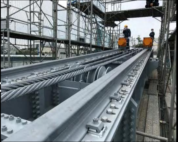
Track Support Beam, Bearing & A150 Rail
