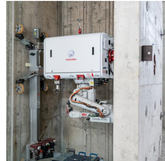
Schindler R.I.S.E Robotic Installation System for Elevators
