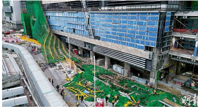
Collapse of a bamboo scaffolding in HK Courtesy of Mingpao News, 13 Jan 2025
