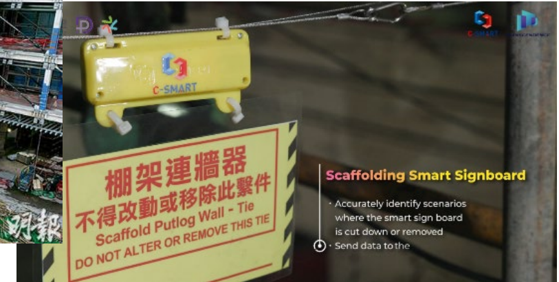
Trial run of digital sensors on scaffoldings at Lamma Power Station (LPS) of HK Electric to enhance scaffolding safety
