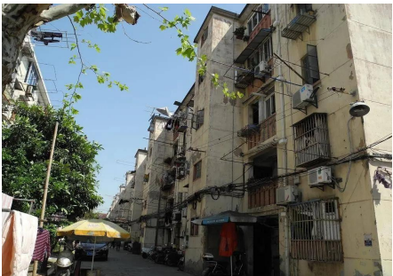
Old Residential Renovation
