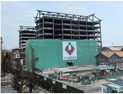
Dilapidated Building Reconstruction
