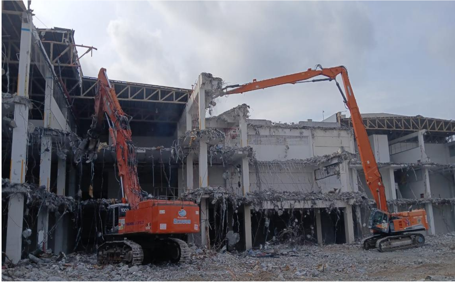
Roof Beam Removal after Rood Slab have been demolished and crushed
