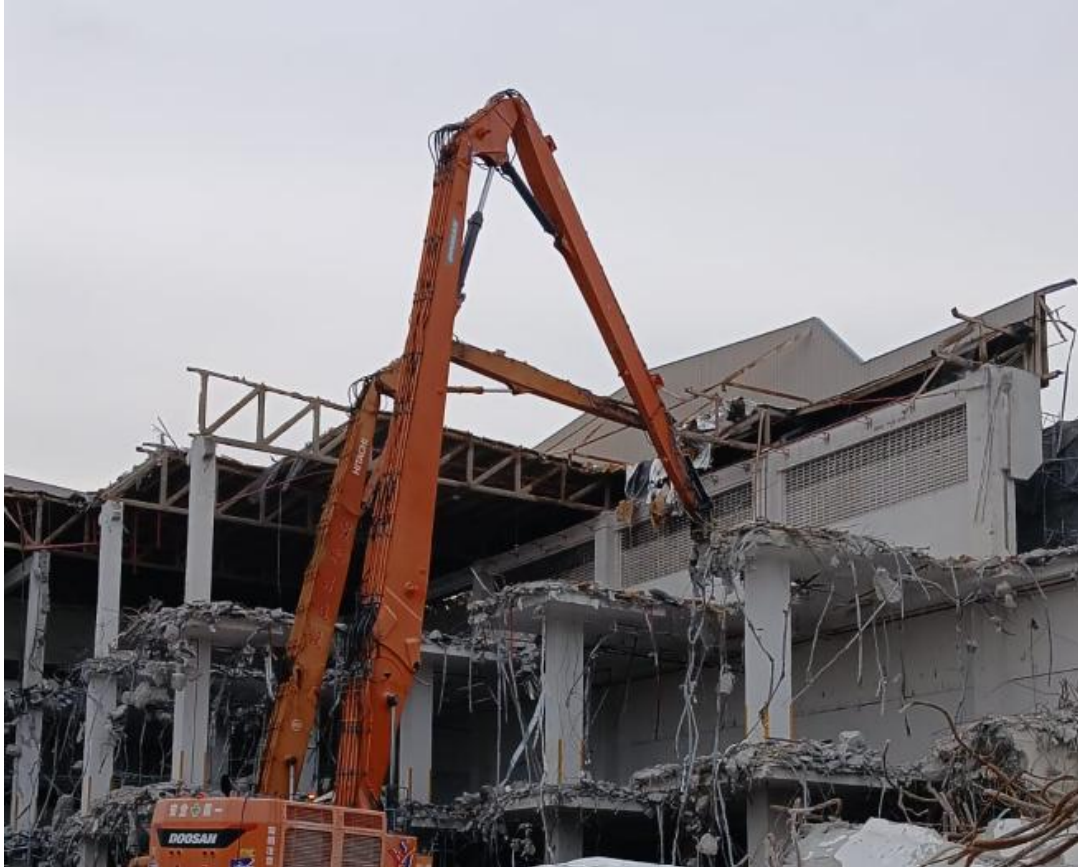
Gable End removal of Façade using 2 ultra long arm excavator.
