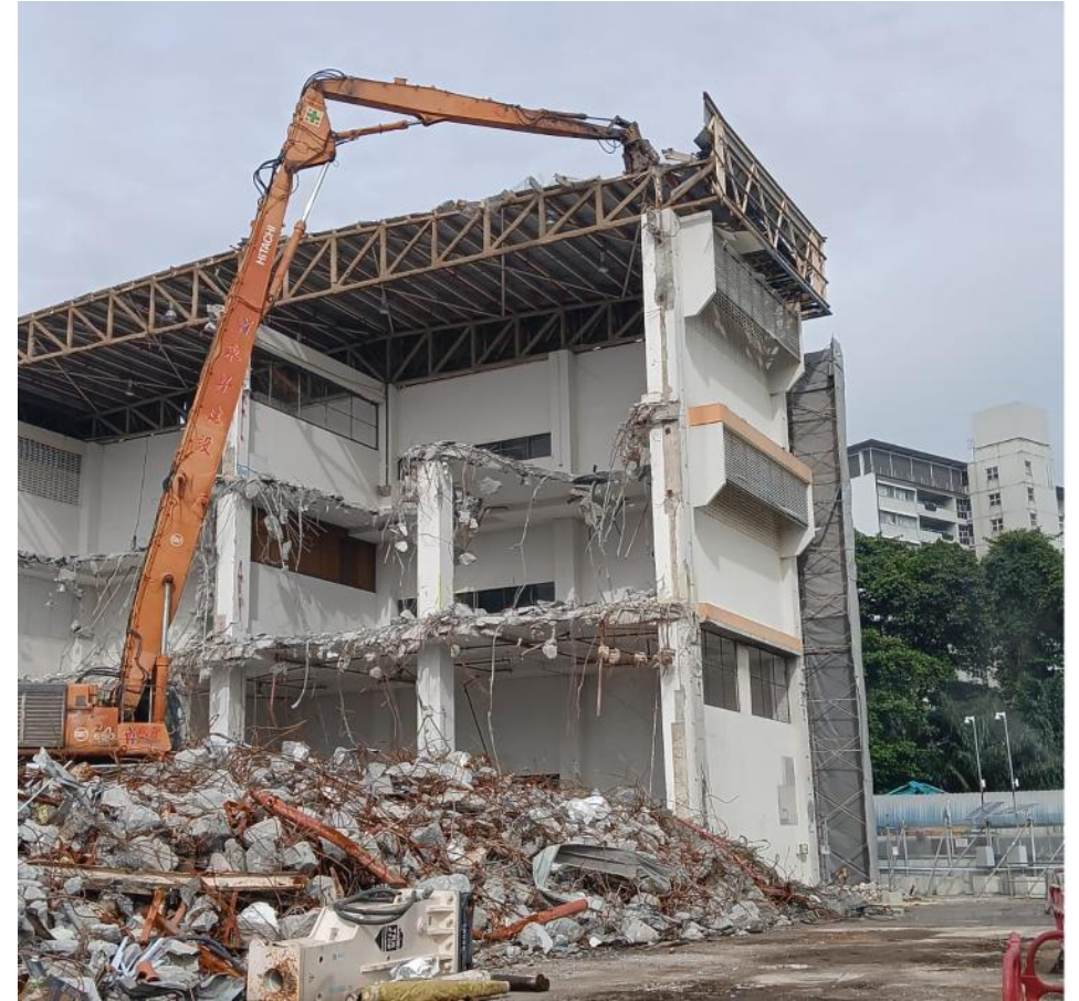
Removal of Roofing sheet and purlins
