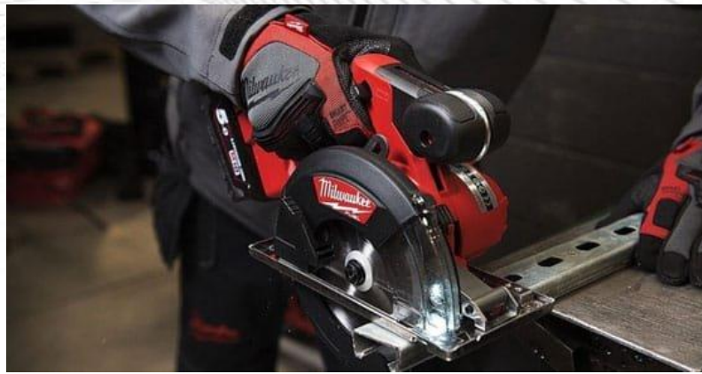
2. Cold Cut to Unistrut
