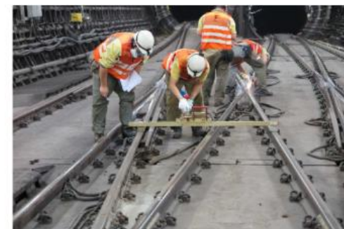
ON-LINE MONITORING AND DETECTION OF RAIL WIDTH TO PREVENT DERAILMENT
