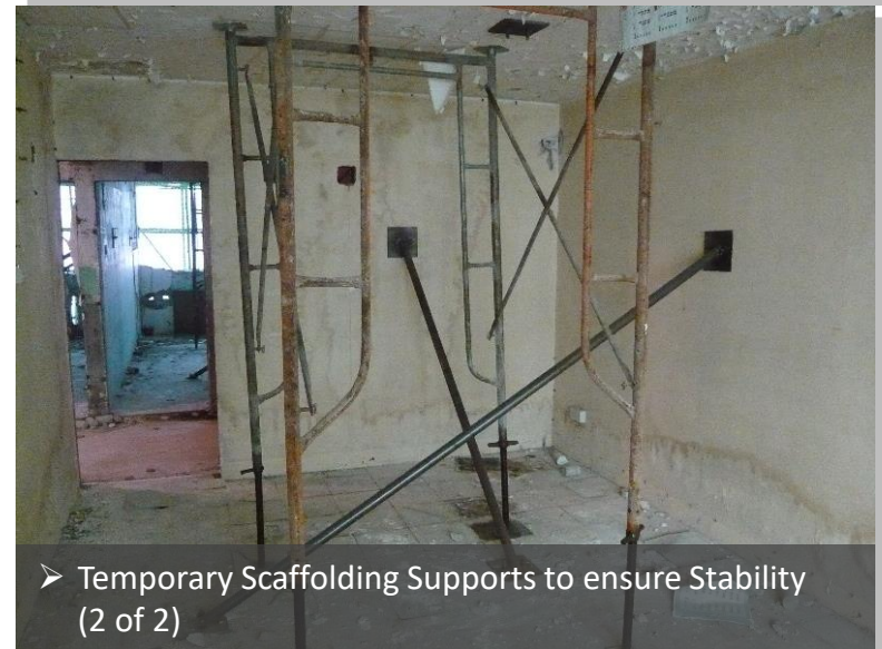
➤ Temporary Scaffolding Supports to ensure Stability (1 of 2)
