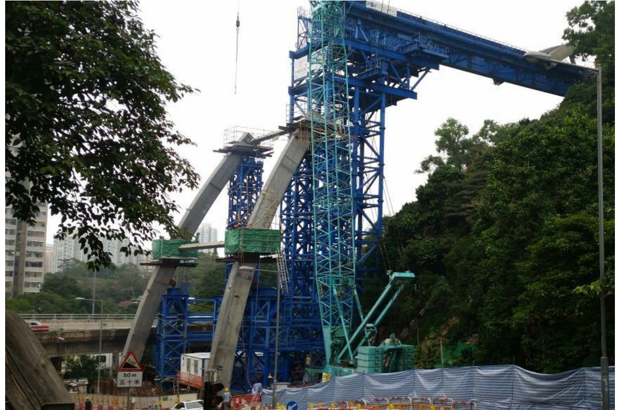
➤ The Photo showing the Erection of Temporary Supporting Steel Structure
