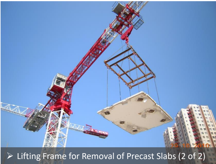
➤ Lifting Frame for Removal of Precast Slabs (1 of 2)
