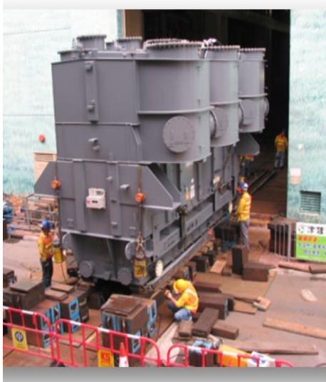
Transformer Erection
