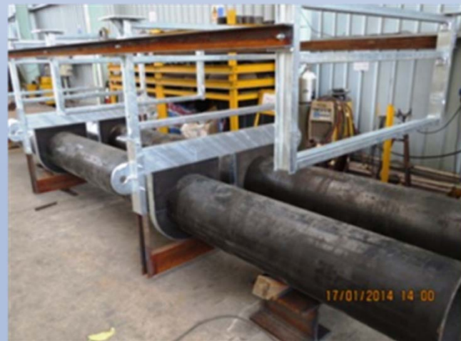
Prefabrication of Pipe Modules
