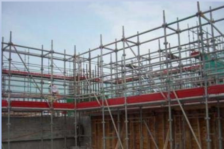
Adequate Guardrails & Toeboards
