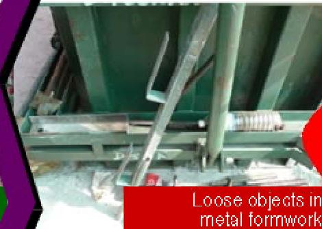
Loose objects in metal formwork
