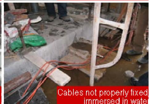
Cables not properly fixed immersed in water
