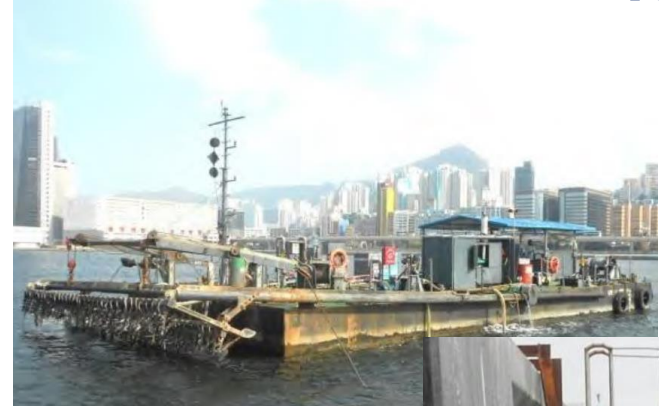
4. Kai Tak Nullah – Reconstruction & Upgrading
