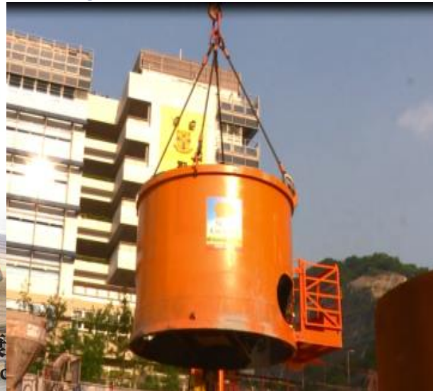
Design to minimize Working at Height e.g. remote control for concrete skip and lifting sheet piles & H piles
