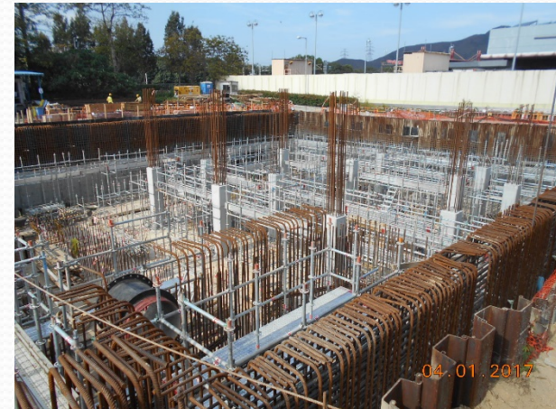
Falsework Erection at Basement
