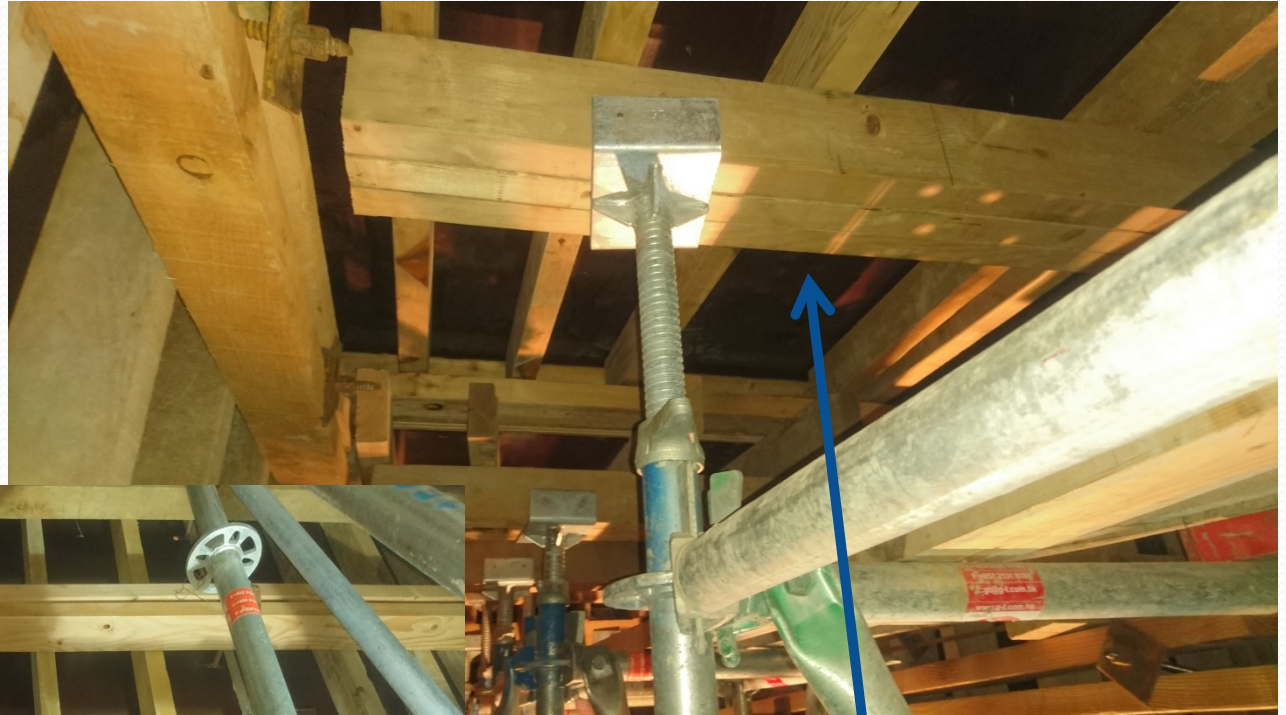
Triple Timber at Joist
