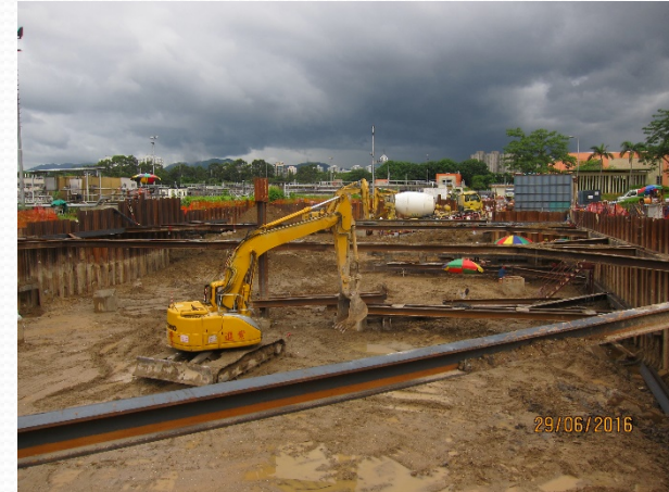
Excavation of Basement
