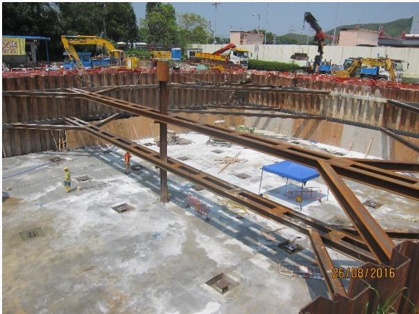
Blinding Layer for Pile Cap
