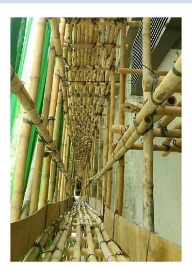
Photo on completed bamboo platform
