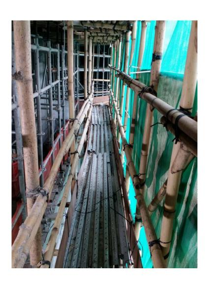
Closely placed bamboo scaffolding with metallic planking
