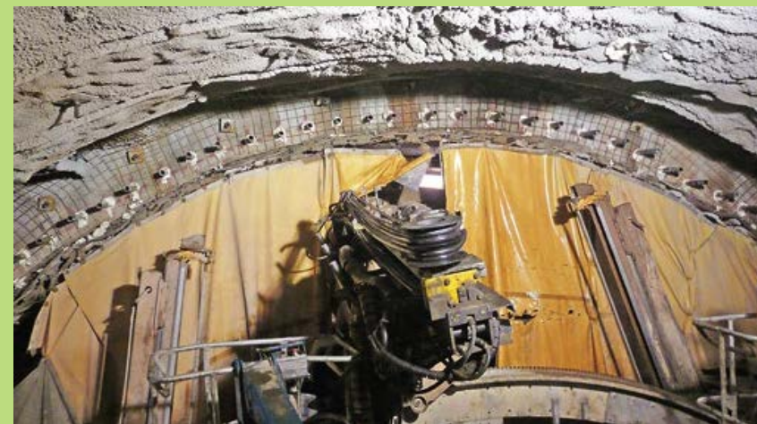
Illustration of complete row of spile bars
