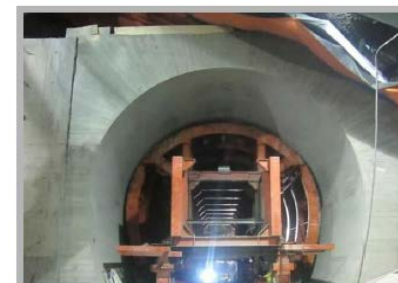
Example of Type 1 & 2 Self Reacting Formwork
