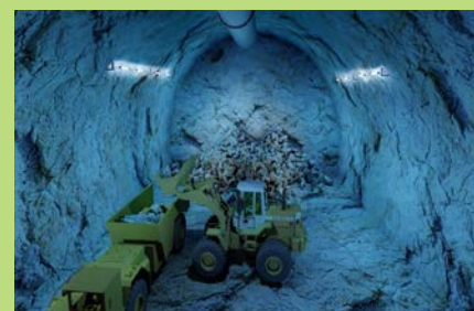
Picture for Full Span Heading Excavation
