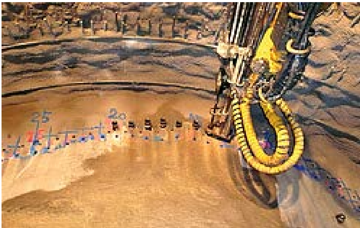
Illustration of spile bars installation
