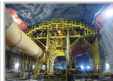
Example of Type 3 Self Reacting Formwork
