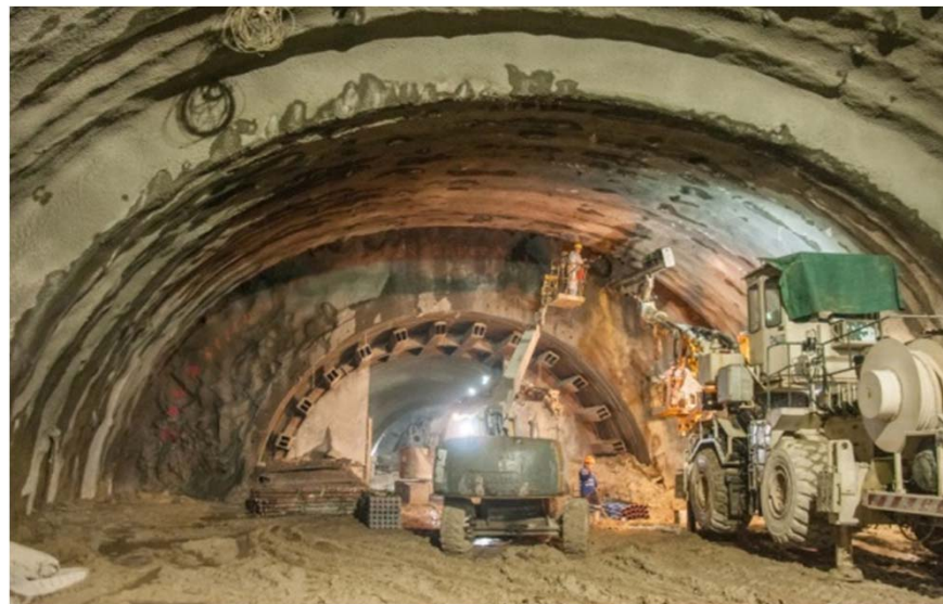
Photo 8 – Temporary Support Installation after each round of excavation and lining dismantling.
