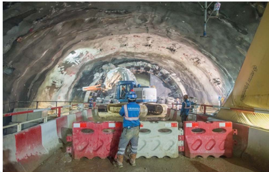
Photo 5 – Enlargement and demolition work face in the upper deck
