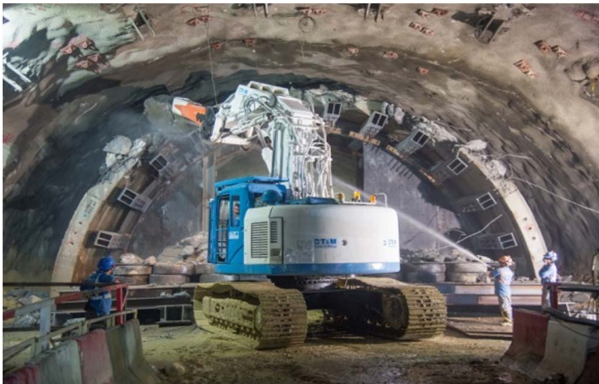
Photo 6 – To avoid overloading the gallery, Segment catching frame and cushions was designed to minimize the impact load. The size of falling segments could be controlled.
