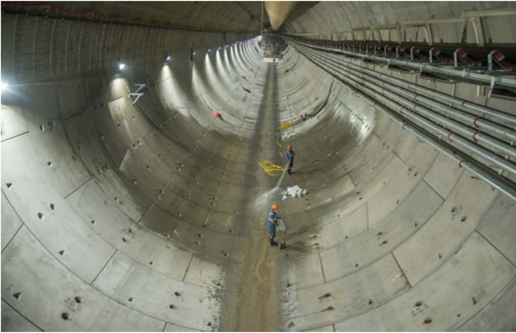
Photo 1 – TBM Segmental Lined Tunnel before Enlargement
