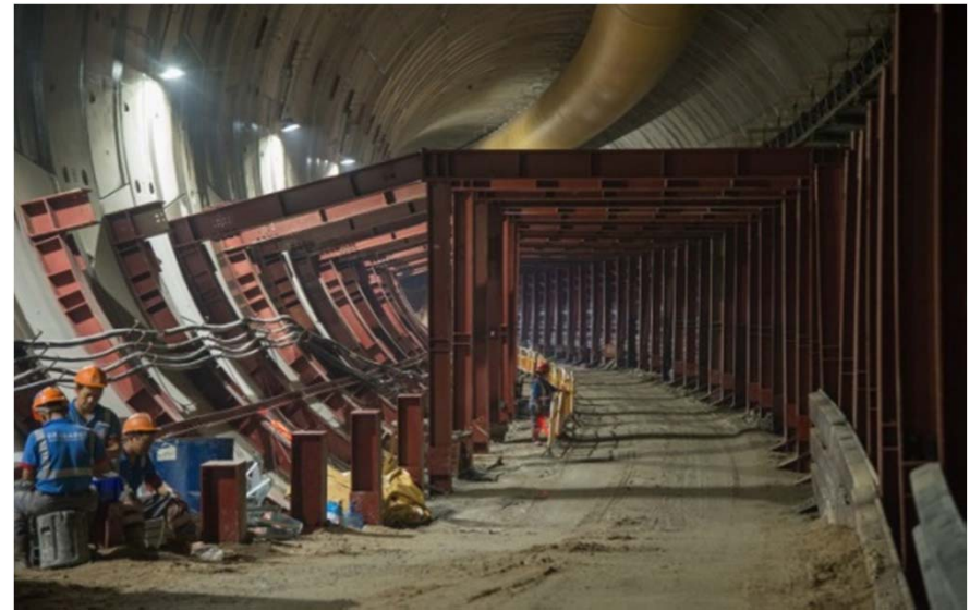
Photo 4 – Steel gallery being erected. It isolates the enlargement and demolition work face, in the upper deck, from the active access road underneath.
