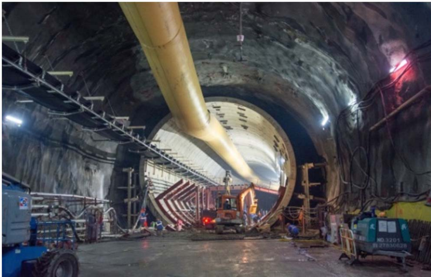
Photo 3 – Steel gallery is being erected inside built segmental lined tunnel
