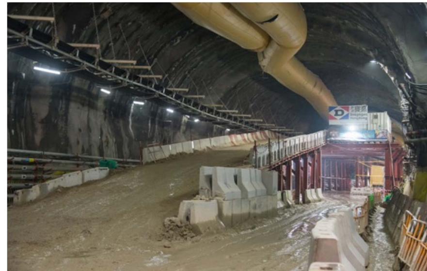
Photo 7 – Access Ramp to connect the enlargement and demolition work face, in the upper deck; and access road underneath to TBM.
