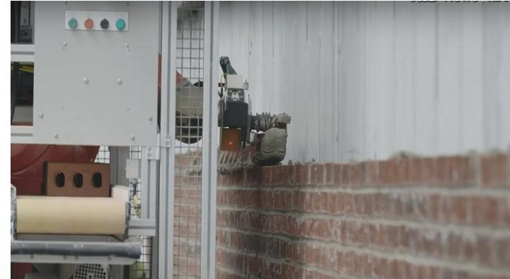
*Bricklaying robot from Semi-Automated Mason*
