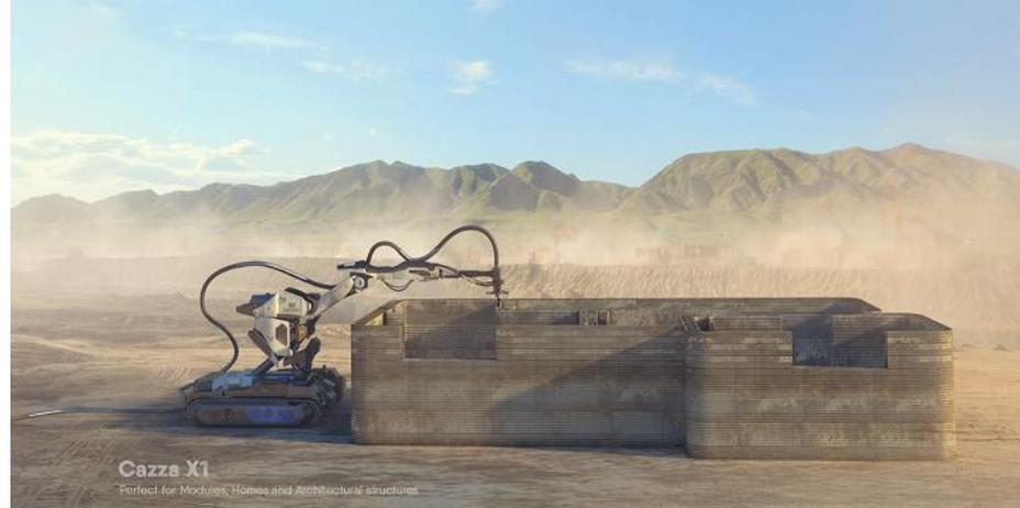
*3D printing construction robot from Cazza*
