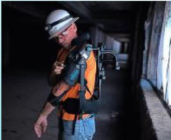
*Upper body exoskeleton to elevates and supports a worker's arms from Ekso Bionics*
