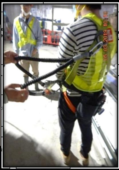
**Length of Lanyard < 1m length shall be used when working on MEWP**
