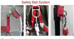
Three different application methods to ensure the worker's safety belt is properly installed
