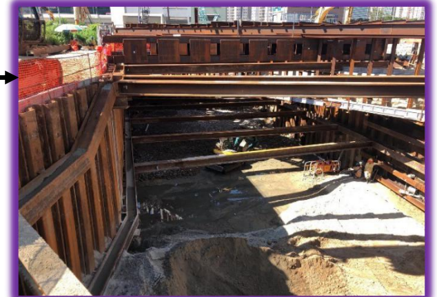
2. Box Culvert Construction at Portion 17
