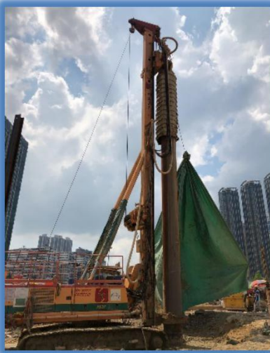
4. Socket H-pile Construction at Portion 1B
