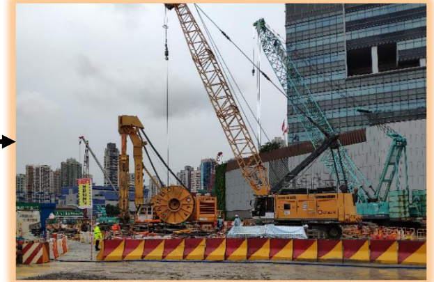
1. Diaphragm wall Construction at Portion 1F and 10
