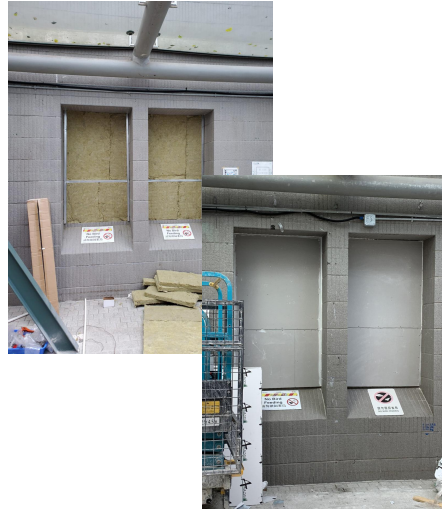
Noise barrier for library.
