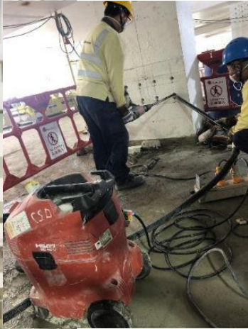
Using vacuum cleaner during drilling works
