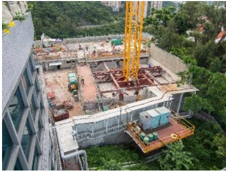
Slab cut from existing structure
