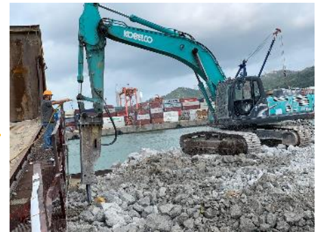
Concrete is broken down to aggregate
